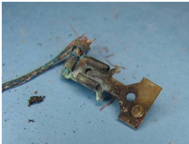
Figure 1: High impedance connection with oxidation
