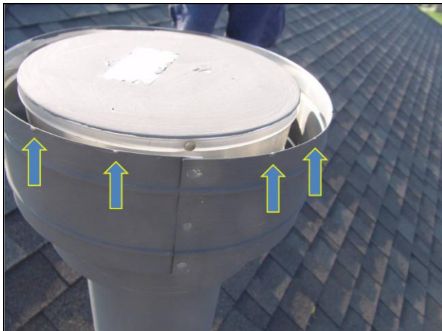
Figure 3: Large surface with multiple discharge points
