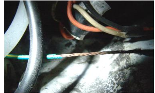
Energized ground from lightning
