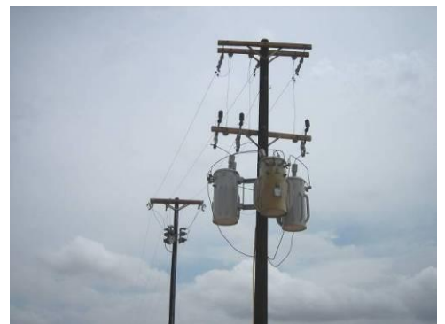
End pole on power line
