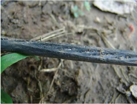
Energized neutral melted insulation
