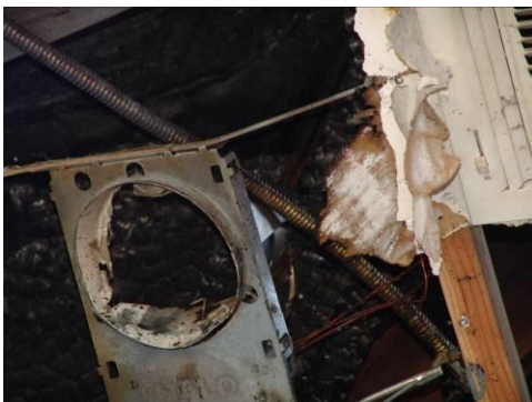
Discharge between CSST and cable
