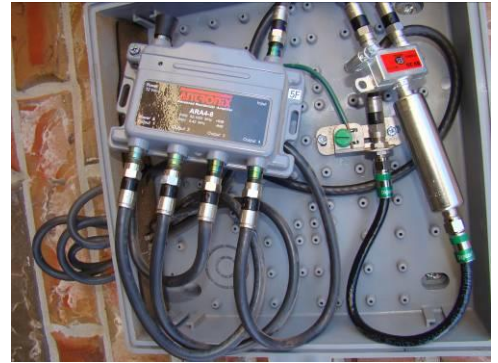
CATV coax grounded
