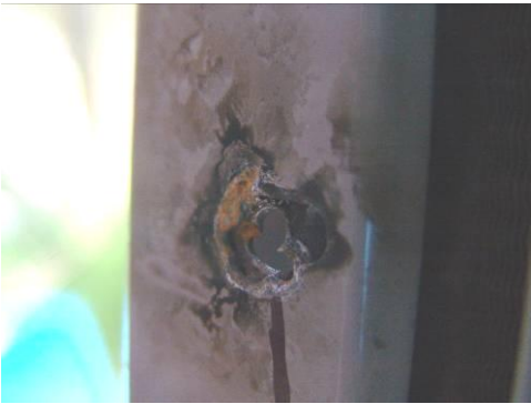
Discharge to bolts on air conditioner
