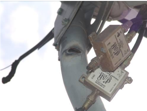
Ungrounded dish with lightning damage
