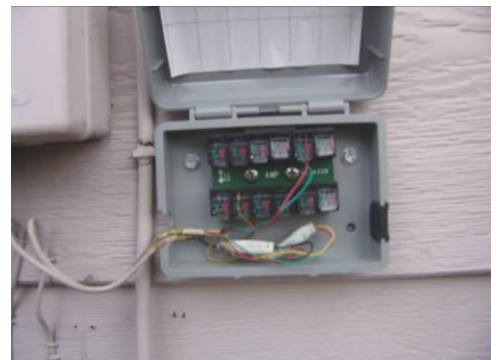
Telephone entrance no ground
