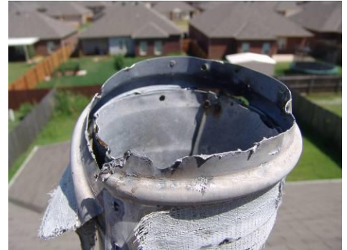
Vent entrance for lightning
