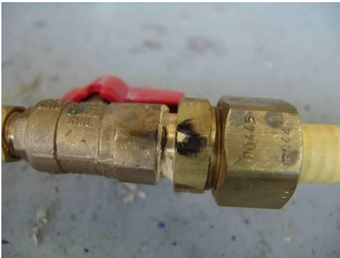
Arcing of lightning on brass gas fitting
