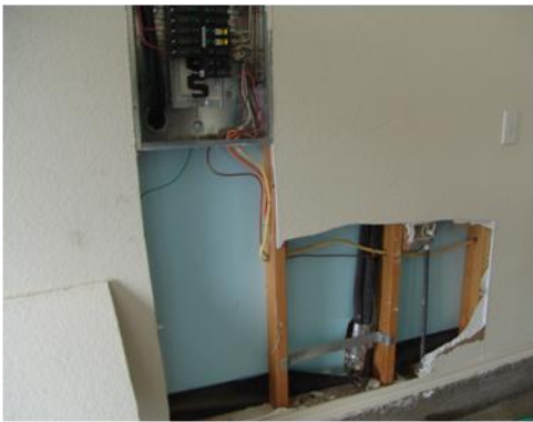
Electrode in concrete
