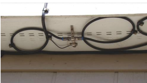
Antenna coax shield connection to ground
