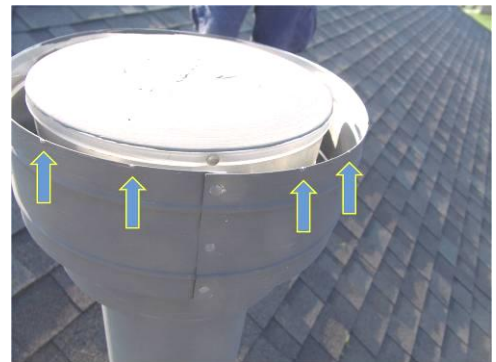
Discharge on edge of metal vent
