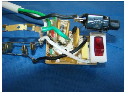
MOVs, circuit breaker, lighted switch
