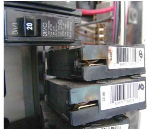
Breaker damage from lightning
