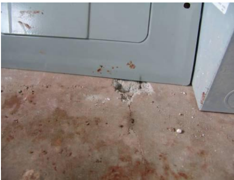
Unbonded rebar arc through concrete
