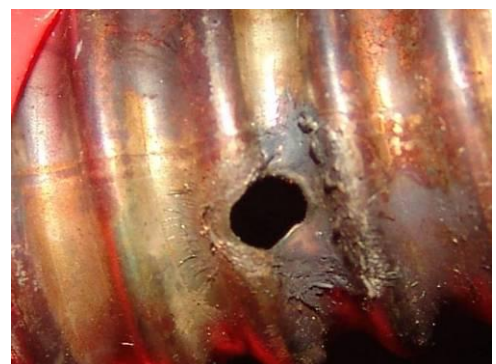
Lightning discharge on CSST
