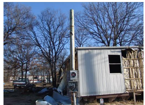
Mobile home service permits 30' to ground
