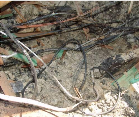
Ungrounded coax discharge to electric
