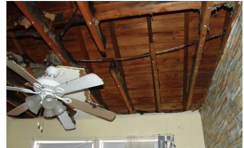
Energized neutral on top of joists
