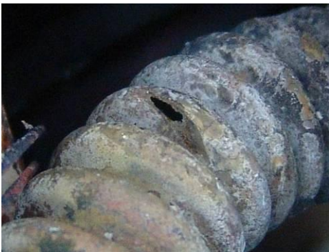
Flexible pipe arc to wiring
