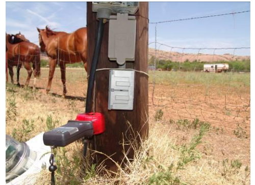
Ground connection utility meter pole
